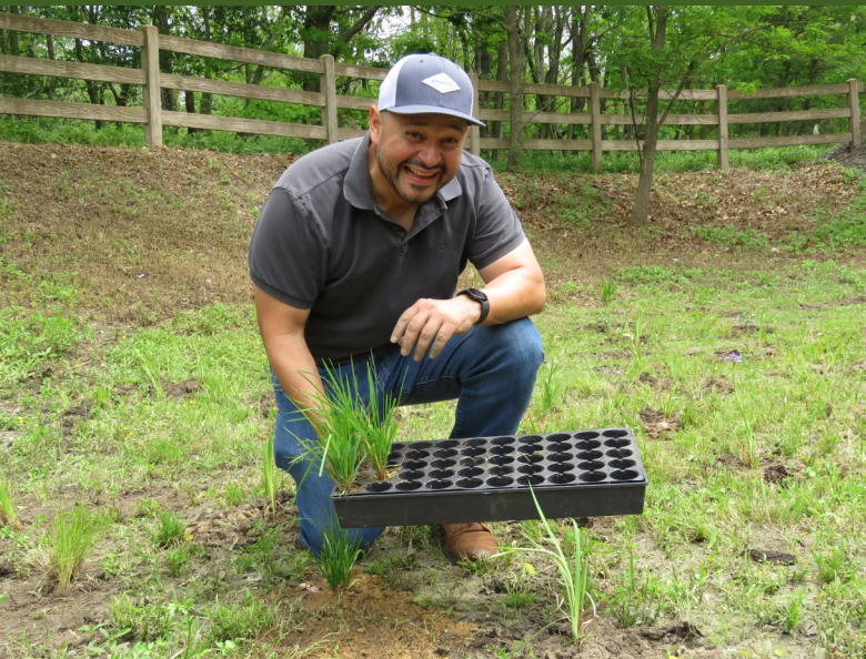
Senior Erosion Control Specialist, Ramon Mejia, installs native plugs in Shemen St. basin, Lakewood Township.
