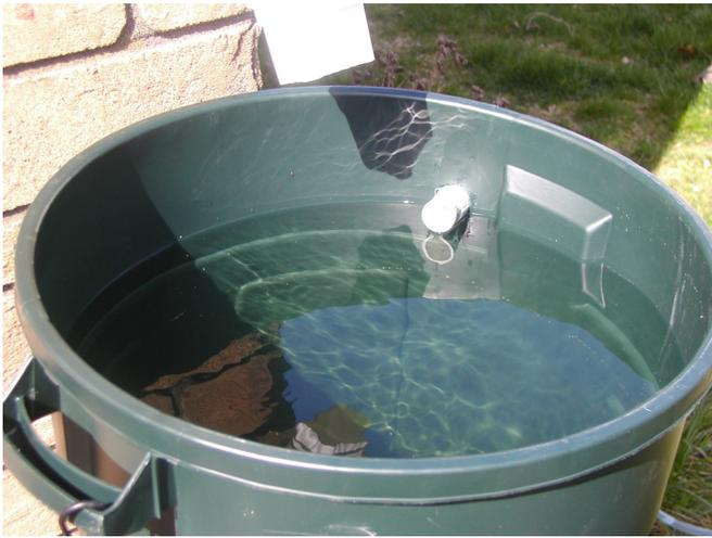
*An example of a rain barrel filled with water. Rain barrels should always be covered with a lid and screen to prevent mosquito infestation.*
