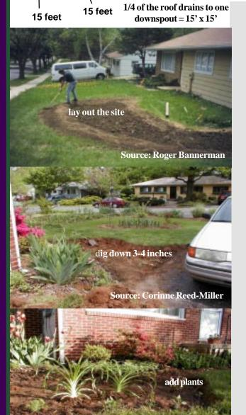
responsible for the bulk of the pollutants in stormwater, a rain garden is designed to temporarily hold water from a one-inch rainstorm, and slowly filter out many common pollutants like sediment, oil, grease and nutrients. Rain gardens require less watering and fertilizer than conventional lawns, and provide habitat for birds and butterflies.
